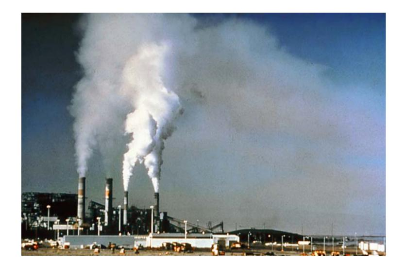
Power plant in New Mexico before installation of flue gas scrubber
