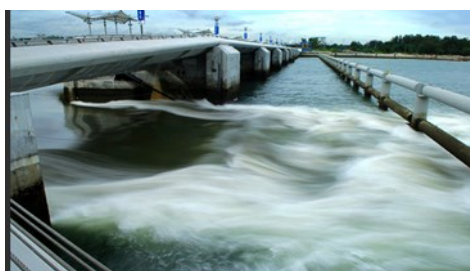
Left: Marina Barrage mechanism, showing diagonally tilted “open” gates. Right: Marina Barrage, with “open” gates; excess water from the reservoir is
